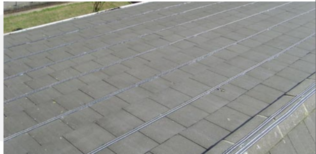
Two rows of track were used butted up to each other on the triangular ridge. The pitch rows were spaced 1m apart.
